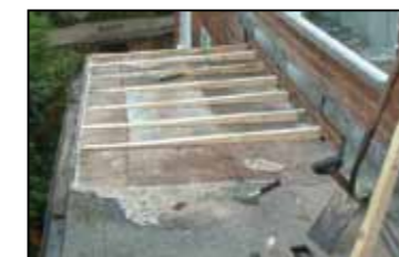
Furrings fixed to a flat roof to aid run-off
