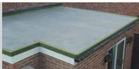
Non-slip finish applied onto topcoat with masked green detail
